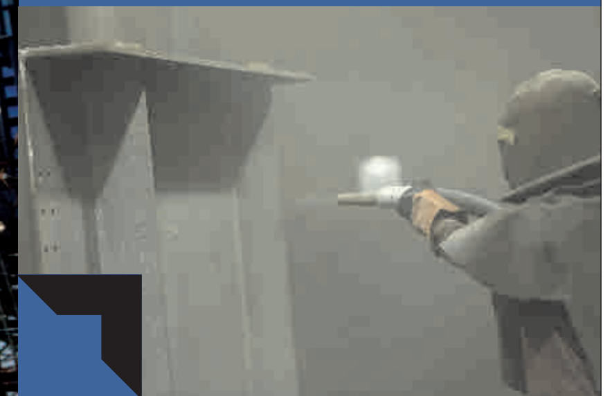
Shot Blasting process
